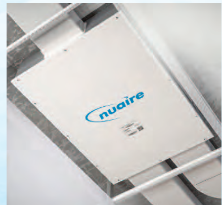
Typical IAQBOX-D installation.
