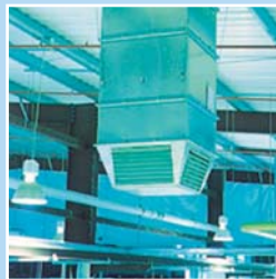
Straight Modular Supply system with high velocity discharge.
