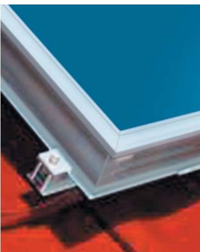
Typical installation of solar unit
